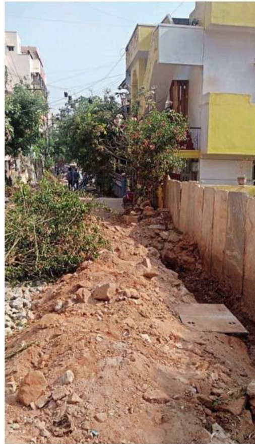
The dug-up piles of debris are kept on the road itself, reducing space for vehicles and pedestrians
