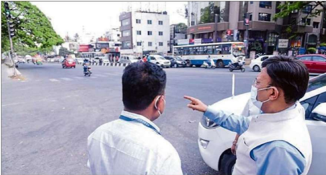
BBMP Chief Commissioner Gaurav Gupta and an official inspect the work on the underpass at Suranjan Das Road on Saturday. SPECIAL ARRANGEMENT
